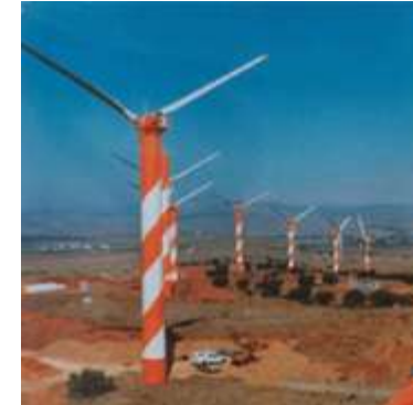
Commissioning of Floda 600 kW, Israel 1992
