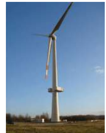
Commissioning of Multibrid 5 MW, Germany 2004
